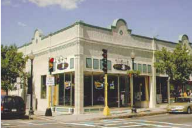
Ten years ago, the historic buildings along Boston's Dana Avenue were nondescript and underdeveloped (top), but the city's 19-district Main Street program has helped renovate them, and public and private dollars have been fostered toward economic redevelopment.
