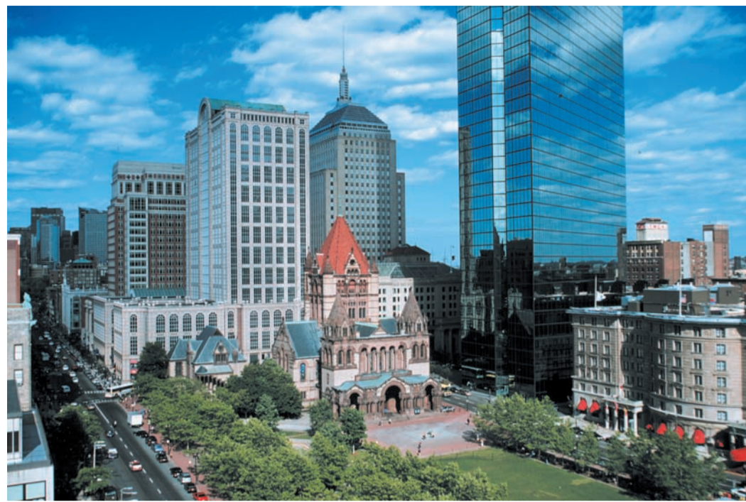
Surrounded by the glass and concrete office towers, Trinity Church is a bastion of traditional design in Boston, presenting a special challenge to the architects charged with rehabilitating – in a sustainable manner – the space for offices and meeting rooms. Photo: Peter Vanderwarker
