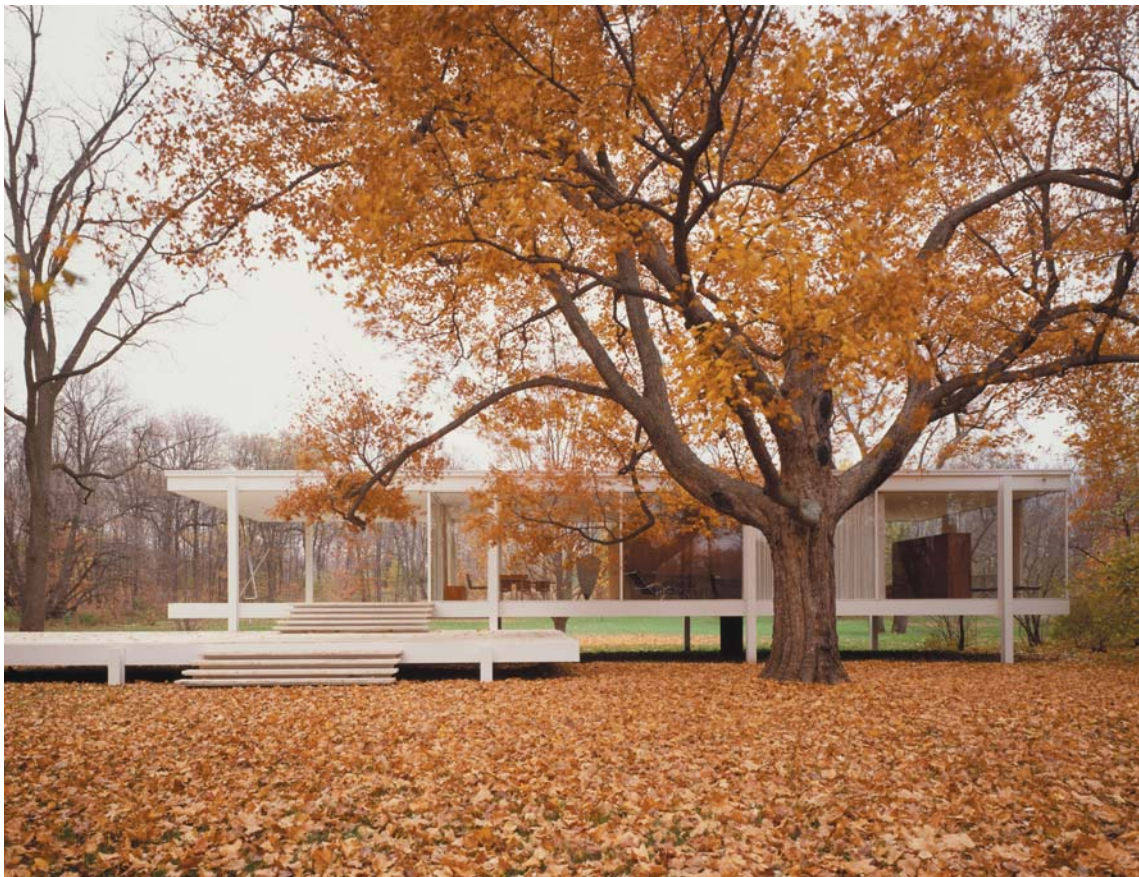
The Farnsworth House – a Mies van der Rohe masterwork – is one of several high-profile Modernist buildings that have been restored in recent years. Now owned by the National Trust for Historic Preservation, the house still needs a roof replacement and repairs to the steel supports and famous travertine steps. Photo: Jon Miller, Hedrich Blessing Photographers; courtesy of Landmarks Illinois
