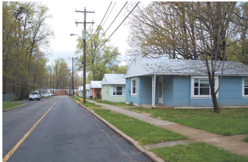
Built between 1948 and 1950, all-steel Lustron houses combined a Modern aesthetic and materials with a pitched roof and low profile that complemented traditional mid-century neighborhoods. Only about 2,500 Lustrons were built nationwide, including 60 at the Quantico Marine Base in Quantico, VA. Today, half of the Lustrons on base have been torn down, and the others shown here face a similar fate. Photo: Kim A. O'Connell
