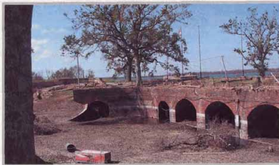
Fort Jackson spent weeks underwater, and tests are still ongoing to determine if its masonry was undermined. Debris and clutter still litter the fort in this recent photo.
